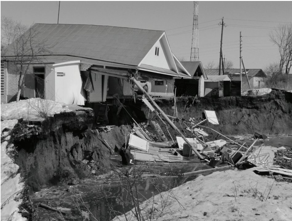
Figure 3. Karst collapse ( d \approx 60 m) in Buturlino (Russia), causing destruction of two residential buildings and a granary in April, 2013.
